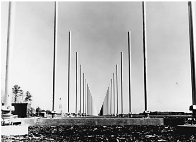
Figure 1.1-17 Very long range (over 1000 nmi) one-dimensional electronically scanned (in azimuth direction) phased-array ROTHR: (a) transmit antenna; (b) receive antenna [1]. (Photos courtesy of Raytheon Company.)
