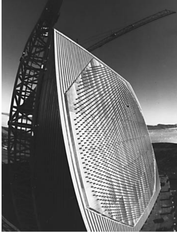
Figure 1.1-11 Upgrade electronically steered phased-array BMEWS in Thule, Greenland [1]. (Photo courtesy of Raytheon Company.)
