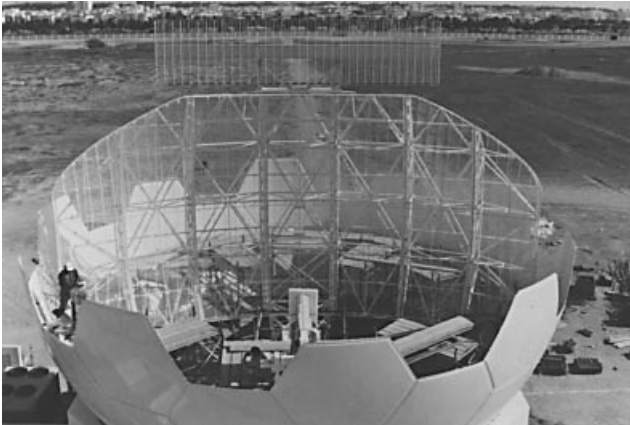
Figure 1.1-6 New fan-beam track-while-scan L-band airport surveillance radar ASR-23SS consisting of dual-beam cosecant squared antenna shown being enclosed inside 50-ft radome in Salahah, Oman. This primary radar uses a 25-kW peak-power solid-state “bottle” transmitter. Mounted on top of primary radar antenna is open-array rectangular antenna of colocated MSSR. This system is also being deployed in Hong Kong, India, The People’s Republic of China, Brazil, Taiwan, and Australia.
