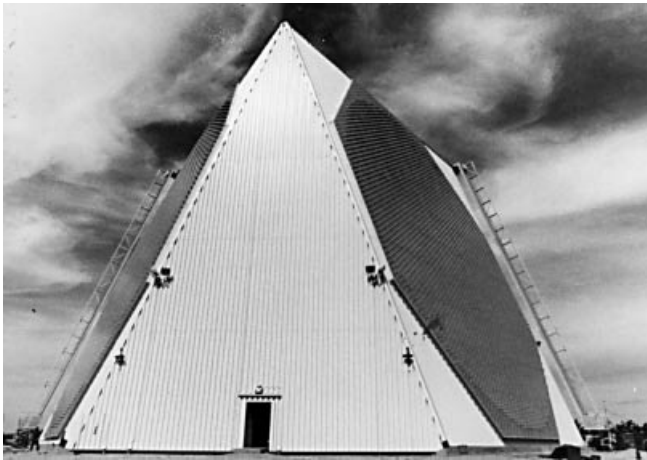
Figure 1.1-14 Multifunction electronically steered two-faced Pave Paws solid-state, phase-steered, phased-array radar [1–3]. (Photo by Eli Brookner.)
