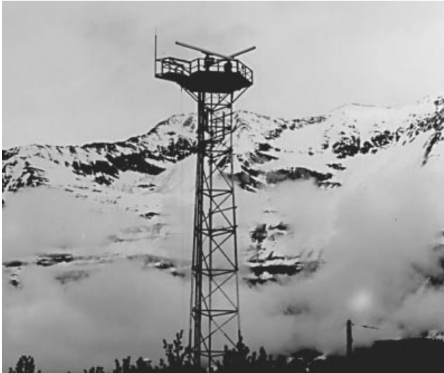
Figure 1.1-3 Fan-beam track-while-scan S-band and X-band radar antennas emplaced on tower at Prince William Sound Alaska (S-band antenna on left). These radars are part of the Valdez shore-based Vessel Traffic System (VTS). (Photo courtesy of Raytheon Company.)
